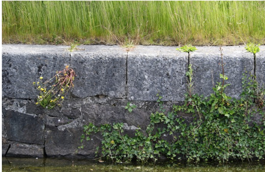
Plate 3: Coping stones on eastern side of canal
